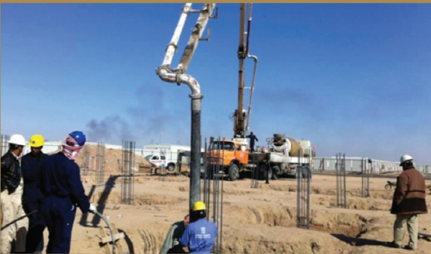
Fire fighting Stations Burgan, North and West Oil Fields – KOC Combained group company – Concrete and Skeleton Work – North Field
